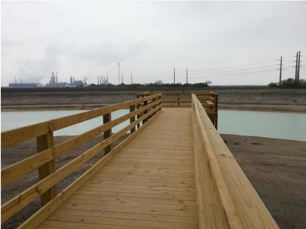
After photo of the finished Overlook/Bench/Crossover unit:
