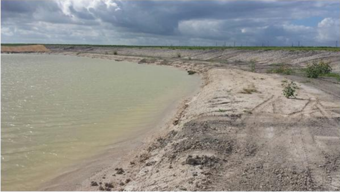
Ground view of project area after pond construction:
