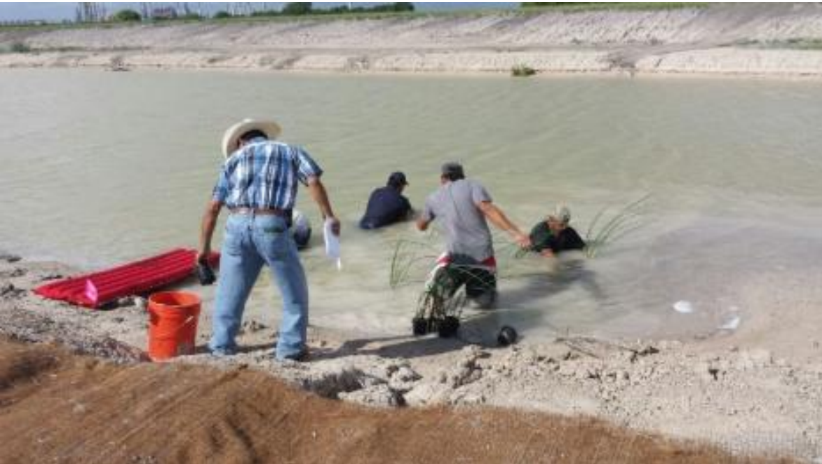
Photo during the planting of the vegetation:
