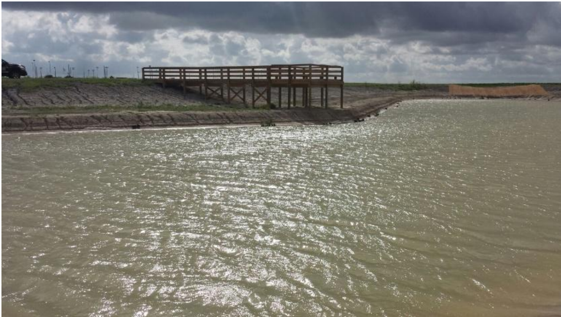
After photo of the finished Overlook/Bench/Crossover unit:
