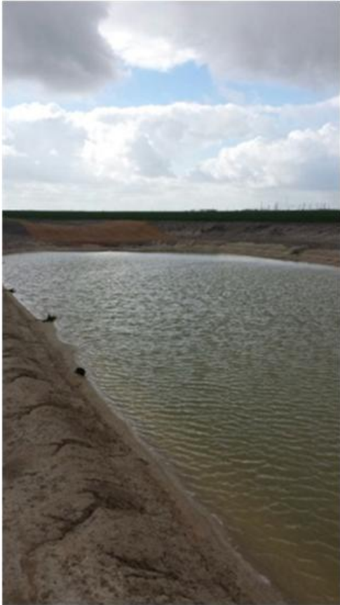
Ground view of project area after pond construction:
